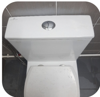
Use of Dual-Flushing Water Cistern
